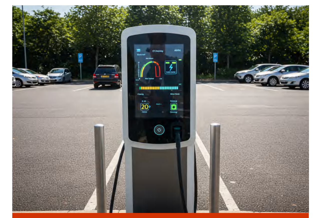
Applying anti-UV ceramic coating on outdoor charging stations.
